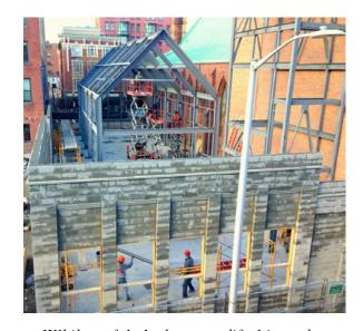
While roof deck sheets are lifted into place with help from a trio of travel-lifts (top center), the perimeter scaffolding comes down since masonry work is essentially complete.
