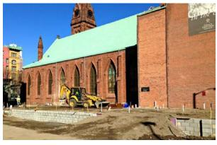
Welcome to the ground floor of The Pavilion at Grace! After skilled masons made quick work of the foundation wall this week, the crew then carried fill material into the void to surround the underground plumbing and rise up to near floor-level. That fill was then carefully compacted in preparation for the imminent pouring of the cement slab that will underlay the final floor.
