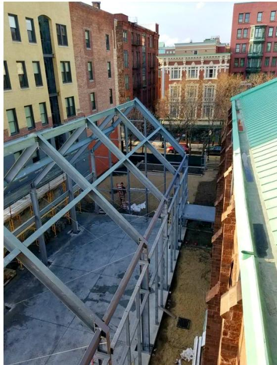
The construction of The Pavilion at Grace made exciting strides this week as the large steel frame for the main gathering space rose rapidly into place.
