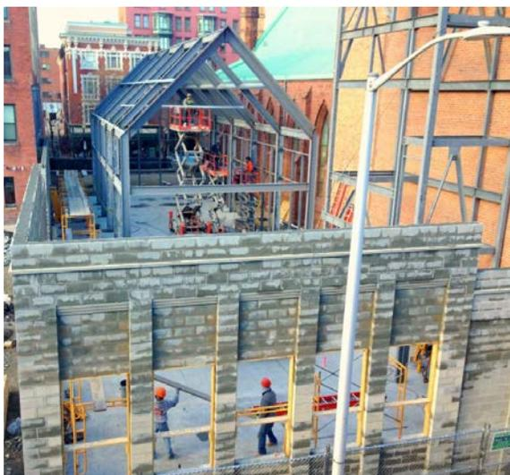
*While roof deck sheets are lifted into place with help from a trio of travel-lifts (top center), the perimeter scaffolding comes down since masonry work is essentially complete.*
