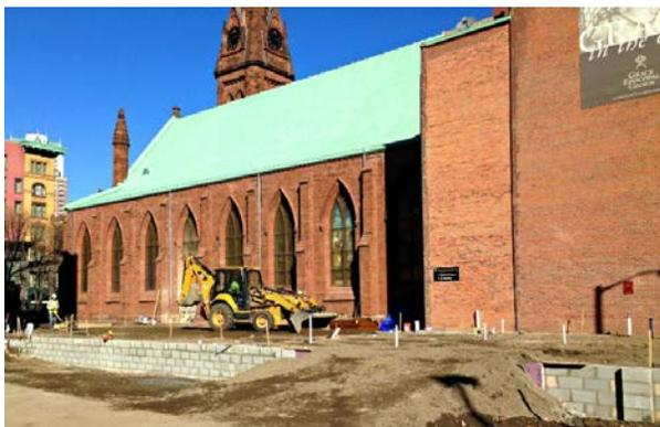
Welcome to the ground floor of The Pavilion at Grace! After skilled masons made quick work of the foundation wall this week, the crew then carried fill material into the void to surround the underground plumbing and rise up to near floor-level. That fill was then carefully compacted in preparation for the imminent pouring of the cement slab that will underlay the final floor.
