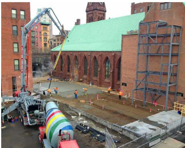
As this week's issue of Grace Abounds hits the wires, a giant pump truck has just finished pouring the entire concrete floor for The Pavilion at Grace. With a crew of workers leveling the material as it pours, and a well-timed sequence of trucks supplying concrete to the hopped of the
