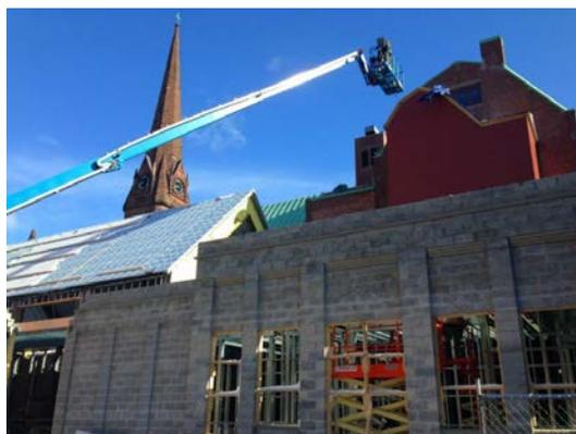
within The Pavilion at Grace), the focus will be upon completing trim work around the perimeter of the roofline (including gutters, etc.) prior to the installation of the final external roofing material. Presently, similar trim work is underway atop the new staitower, with that structure expected to be fully enclosed very shortly.
