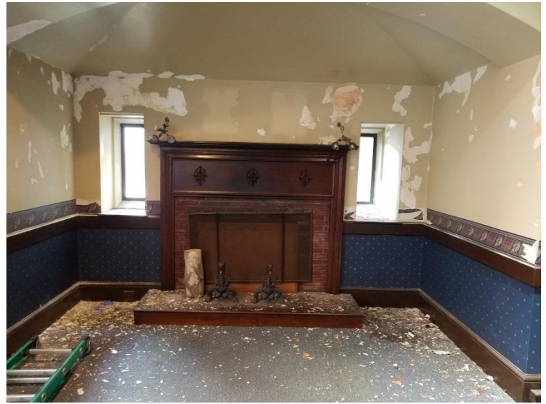
The Chafee Room Fireplace Nook (prior to renovation)
