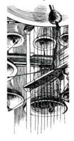
first rung on Easter Day, March 31, 1861. The bells, cast by Henry N. Hooper & Co. in Boston in 1861, are placed in two decks in the tower. Their aggregate weight is 8 tons, and their original cost was approximately \$6000. The bells are unusual in design and character in that they were founded on the proportion of the Spanish bell, which is longer in the waist and gives the minor third in the harmonics instead of the major third that is more commonly used.
