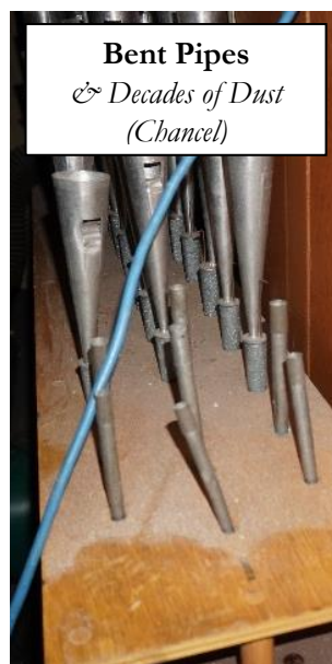
Pipes collapsing in on themselves (Chancel)
