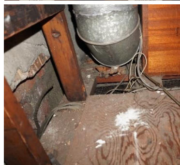
Pipes stopped off with felt (Chancel)
