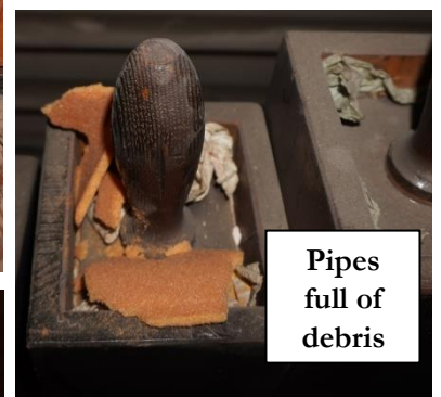
Pipes stopped off with felt (Chancel)
